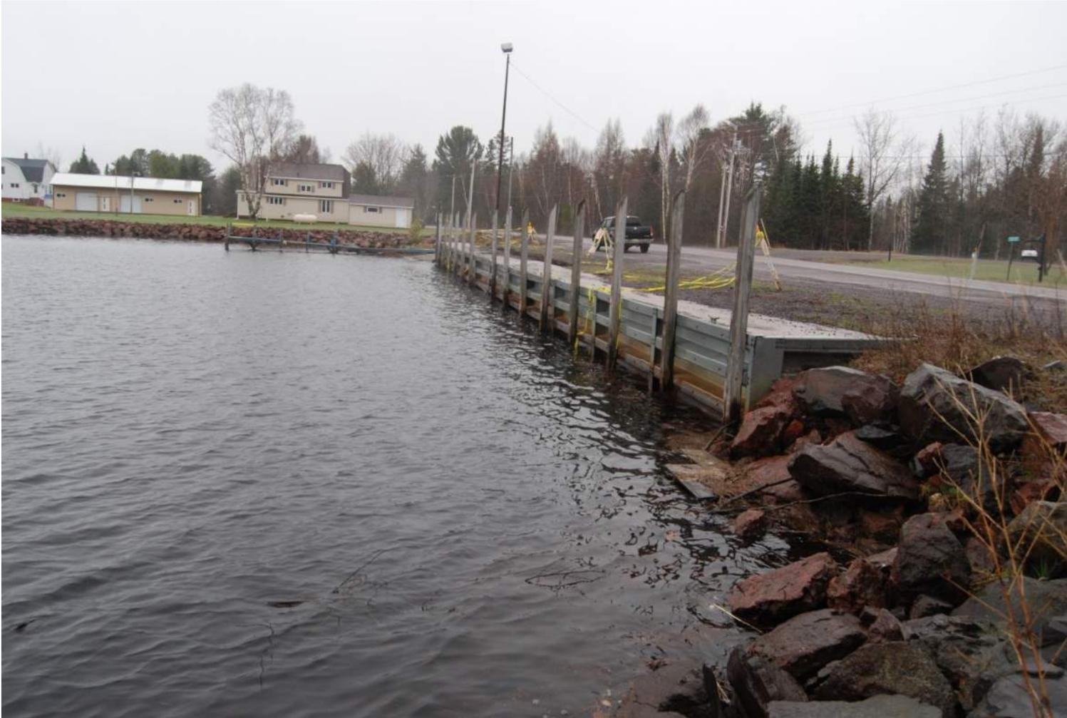
Eventually the bin wall at the boat launch will need to be replaced as the bottom of the existing steel wall begins to rust out. The Township is interested in applying for grant funds to assist it replace the wall. In addition, the Township wishes to make
